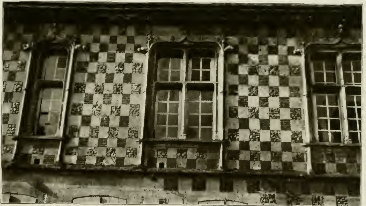
PLATE 166. Detail, house at Verneuil, Eure
